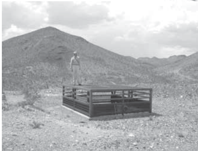
THE AUTHOR checks one of the many bat gates—many of them ornate—that he has designed for abandoned mine openings over the past 16 years.
